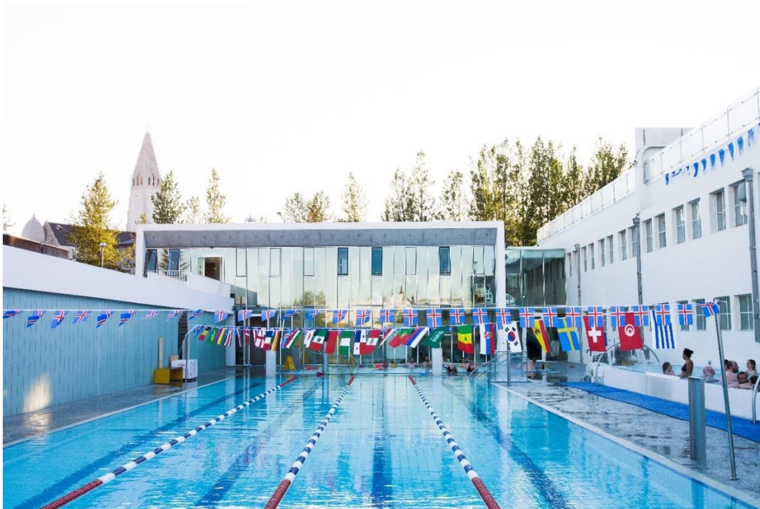
Swimming pools and bath houses are common in Iceland and it is important that they are accessible to all. This old Swimming pool in the neighbourhood of Sundhöll was rebuilt with a new accessible pool area. Photo: City of Reykjavik
